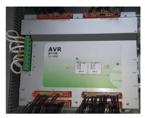
The AVR Z110 automatic voltage regulator is designed as a single-board module and contains:
